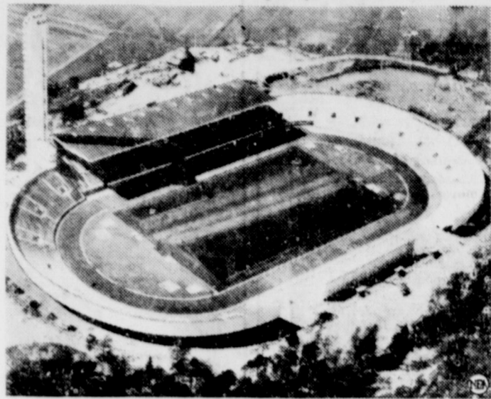
This aerial view of the stadium in Helsinki presents a scene of inactivity, but 60,000 people will fill it every day to watch the cream of the world's athletes perform in the 1940 Olympic Games. A second deck is being added to the structure.
