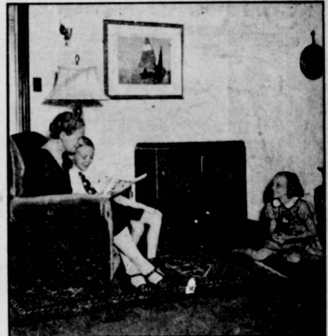
This sample photo shows a vented circulating gas heater in the home of one of our customers.
