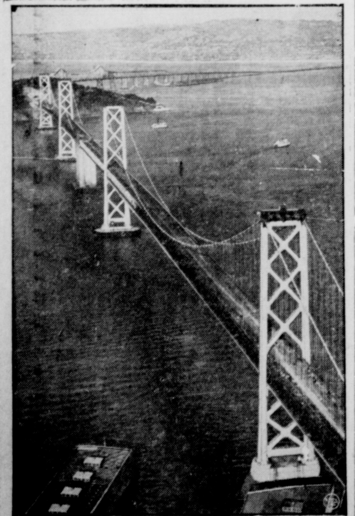
Completed except for minor details, the San Francisco-Oakland Bay bridge, stretching 4 1/2 miles across San Francisco bay, is seen here, ready for its official opening, Nov. 12. This $77,000,000 bridge, largest in the world, was built to carry six lanes of autos on the upper level and trucks and railways on the lower level. As the span crosses Yerba Buena Island, left center, it passes through the world's largest bore tunnel. This view looks from the San Francisco side toward Yerba Buena Island and Oakland and Berkeley in the distance.
