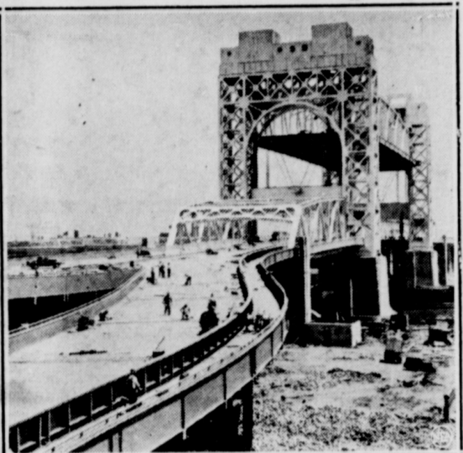
A motorist's-eye view in this picture of the Manhattan approach to New York's gigantic Tri-Borough bridge. Straight ahead is the drawbridge across the East River, one of the series of spans that comprise the vast project linking Manhattan, Bronx and Queens.
