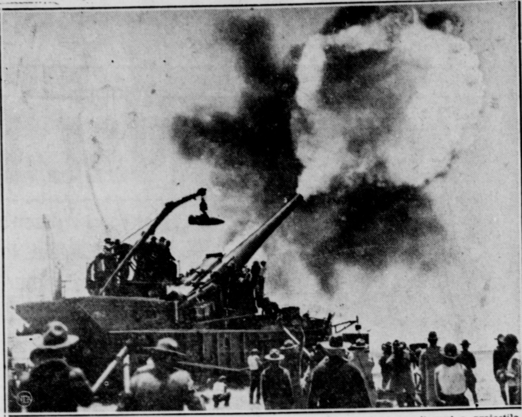
With earth-rocking repercussion, this huge 14-inch railroad rifle is shown as it sent a projectile screaming through space toward targets 26 miles distant, in tests along the California coast. Simulating war-time conditions, the scene of the firing was near Don, Calif., about 40 miles north of San Diego. So terrific is the shock of firing the guns, which propel a 1400-pound shell, that they have not been used since 1928. Windows in coast houses for miles around then were broken by their discharge and many Californians believed an earthquake was in progress.
