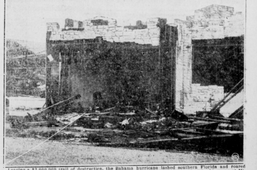
Leaving a $3,000,000 trail of destruction, the Bahama hurricane lashed southern Florida and roared into the Gulf of Mexico at a 130-miles-an-hour clip. The havoc wrought is evident in this scene at Miami Beach, where store fronts were blown in and roofs stripped from many buildings.
