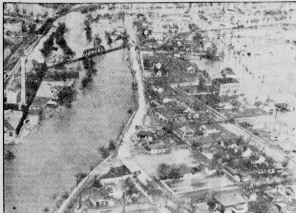
Flood waters surging far over the banks of Black river spread devastation over Poplar Bluff, Mo., this airview showing a section of the city where water was from three to seven feet deep in homes and public buildings. More than 800 families were removed from their homes as the danger increased and refugees were housed in buildings on higher ground, food being provided by FERA funds, with the Red Cross also aiding. More than 100 boats piloted by militiamen patrolled the area.
