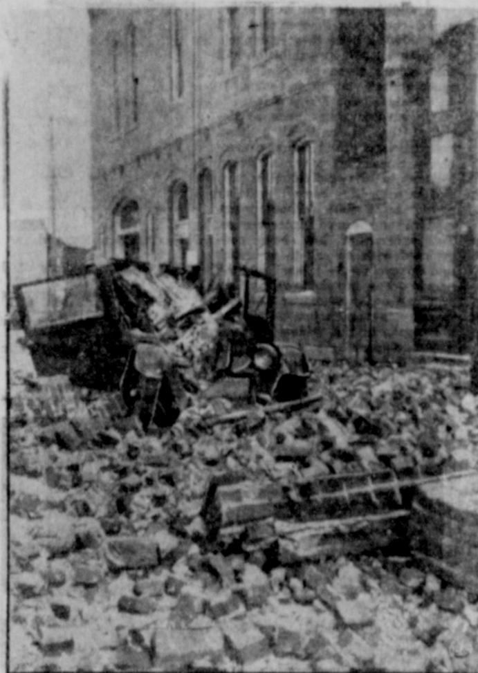
Size of the reconstruction task facing Helena is indicated by this picture, a scene of ruin along one of the capital's main streets, damaged heavily by the recurrent quakes. An automobile parked near the stores is seen after an avalanche of bricks had plunged down on it from business structures in the latest series of shocks that made thousands flee the city.
