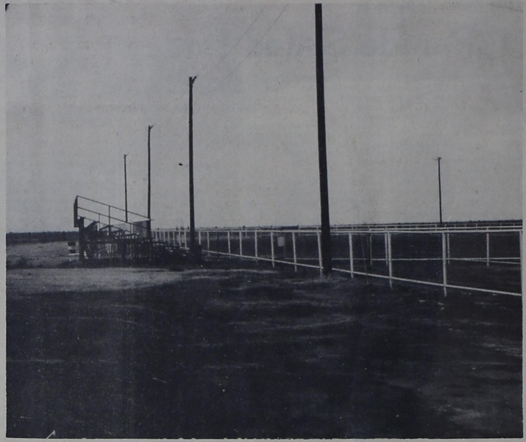
NEW ARENA READY --- Bovina's new roping arena will be put into use for the first time during the Bull Town Days celebration which begins tomorrow (Thursday). Constructed this summer by members of Bovina Roping Club, finishing touches
