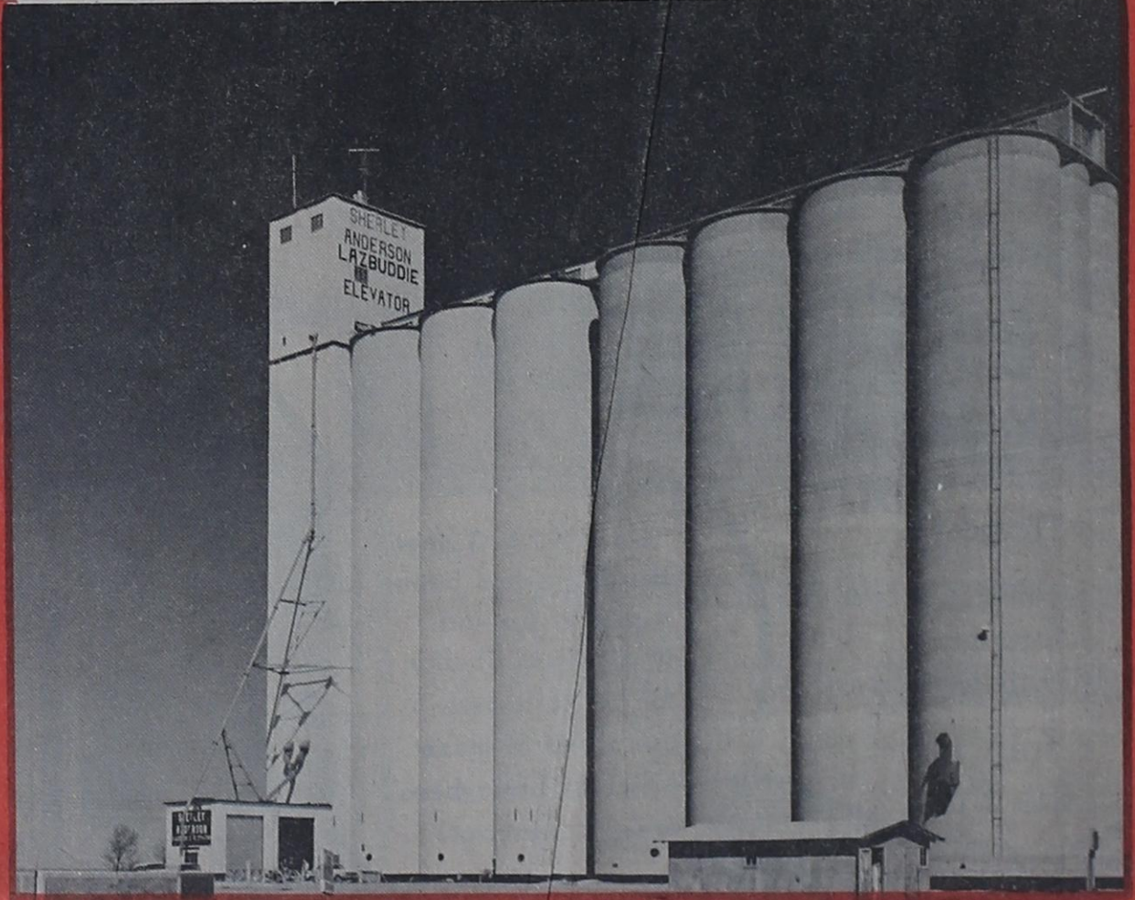
Sherley - Anderson LAZBUDDIE ELEVATOR
