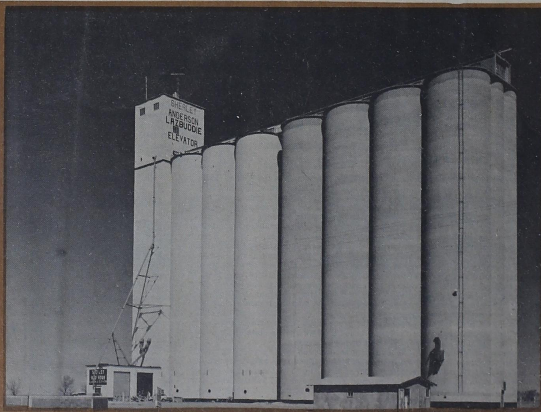
Sherley - Anderson LAZBUDDIE ELEVATOR
