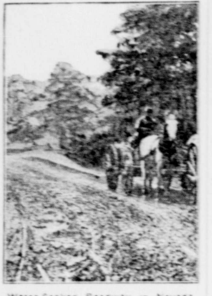
Water-Soaked Roadway in Nevada.
