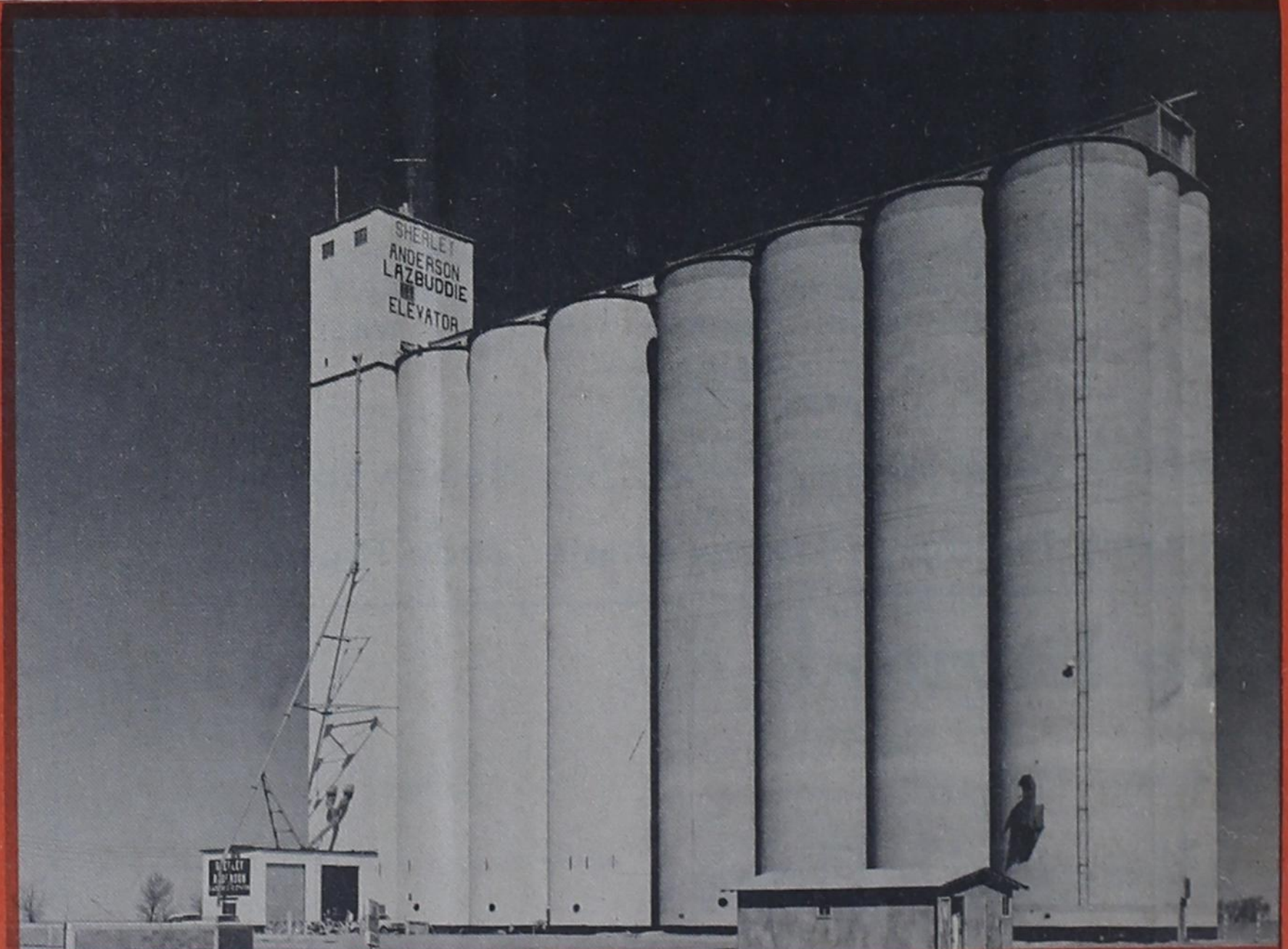
Sherley - Anderson LAZBUDDIE ELEVATOR
