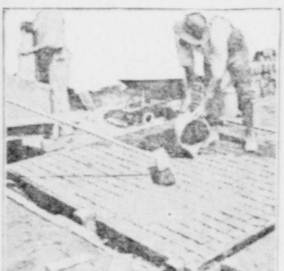
Laying Brick Pavement.
