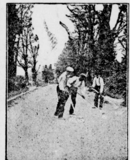
Making Necessary Repairs on Macadam Road.
