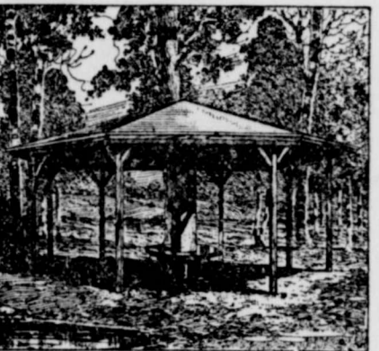
Picnickers Have Little Fear of Passing Rainstorms When a Substantial Shelter is Near to Protect Clothing and Food.
