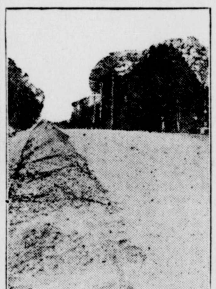
Water Drains Readily From This Type of Highway.
