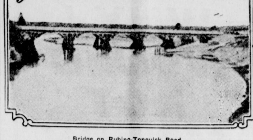
Bridge on Rubino-Tonguisik Road.
