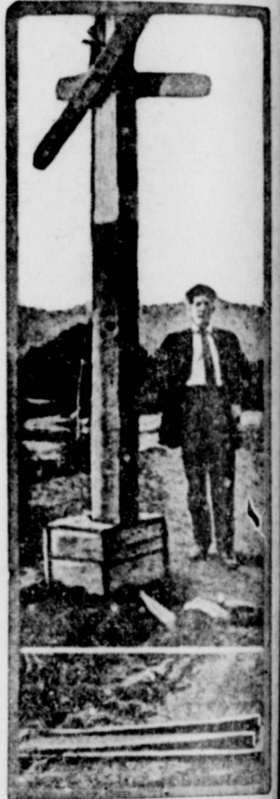
Highway Block Signal and the Trap at the End of the Dangerous Street Which Operates It.
