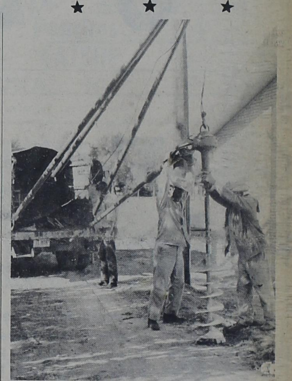
MORE CONSTRUCTION -- Workmen are shown drilling a post hole to be used by the new cable TV system which is being installed in Bovina. The system is expected to be completed in about two months, according to T. M. Monk, who is helping with the installation here. Holes for the posts which will support the cables are now being dug throughout the town. "When the system will be ready for use depends on how fast needed equipment arrives," Monk says.
