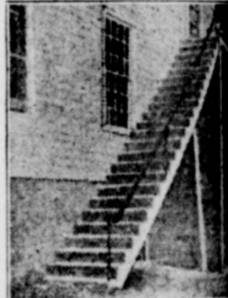
By Constructing the Outside Staircase of Concrete, a Dependable Fire Escape Was Provided at a Small Cost.
