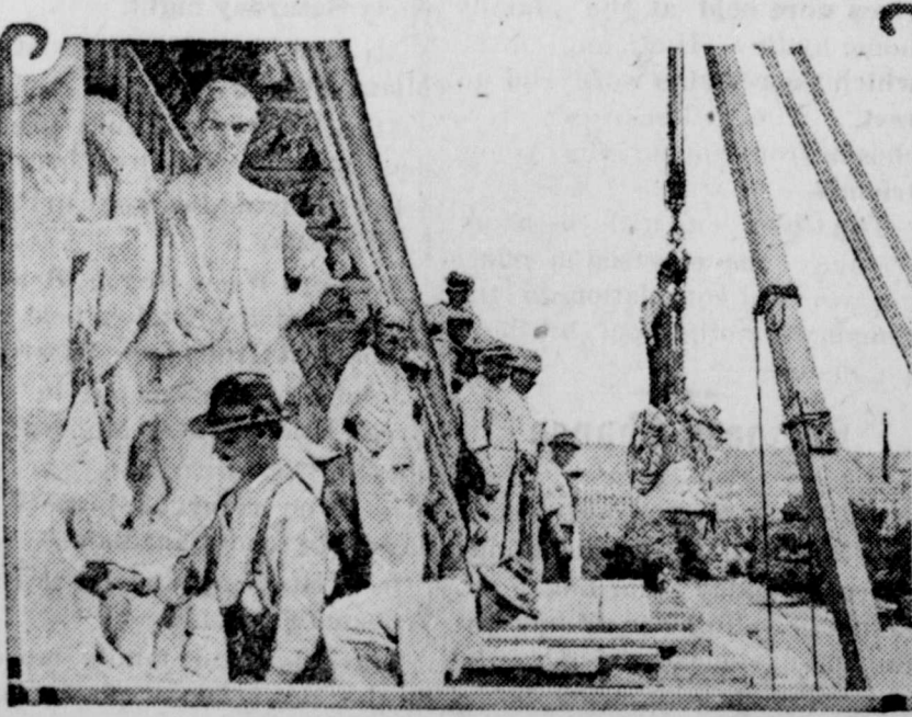
The laying of the final stone shown in the photograph completed the construction of the national capitol, which for more than 50 years has been unfinished. This was the last step in the construction of the pediment of the east wing of the house of representatives, a companion piece to the pediments over the main entrance and the senate wing. This portion of the house wing has been blank since the wing was nominally completed in 1857. An appropriation of $75,000 in 1908 provided for the final work of construction. This final pediment has been constructed by Paul Bartlett, who calls the design "The Democracy of the United States as Expressed by the Types of the Working People."
