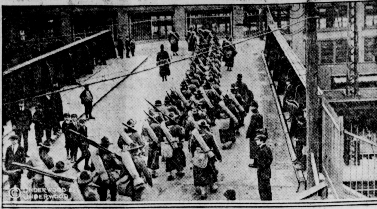
Militia of the New York National Guard crossing a bridge at Hastings-on-Hudson to enter and guard the plant of the National Conduit and Cable company, because of the fight between the strikers, former employees at the plant, and the directors, who refuse to advance the wages of the men.
