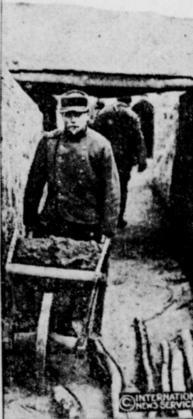
One of the deep trenches on the firing line in northern France. The allies have constructed hundreds of miles of ditches like this.
