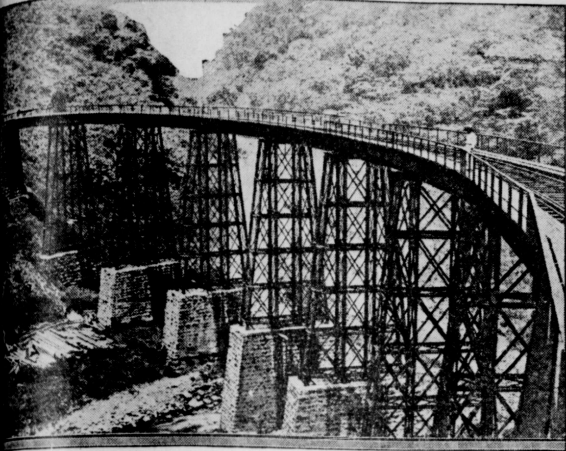
This is one of the two bridges on the line of the railway from Vera Cruz to Mexico City, the control of which is so much to the success of the American troops. The bridges are only a few miles from Vera Cruz, and their destruction would seriously hamper the movement toward the capital.
