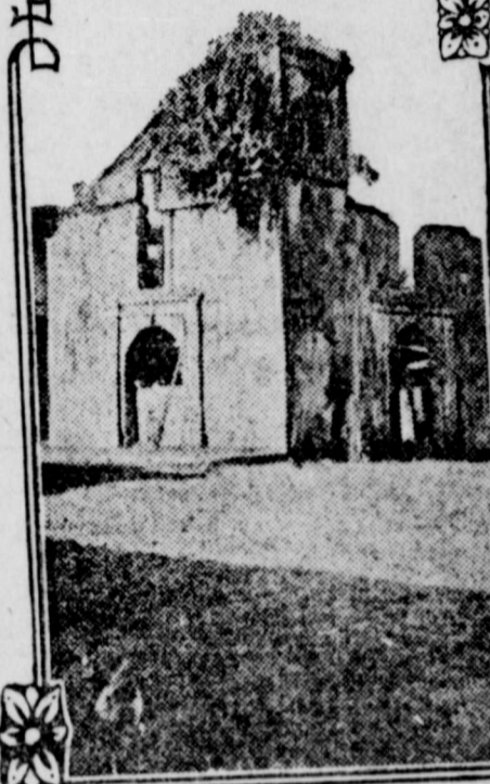
Remains of The Old Church at Porto Bello.
