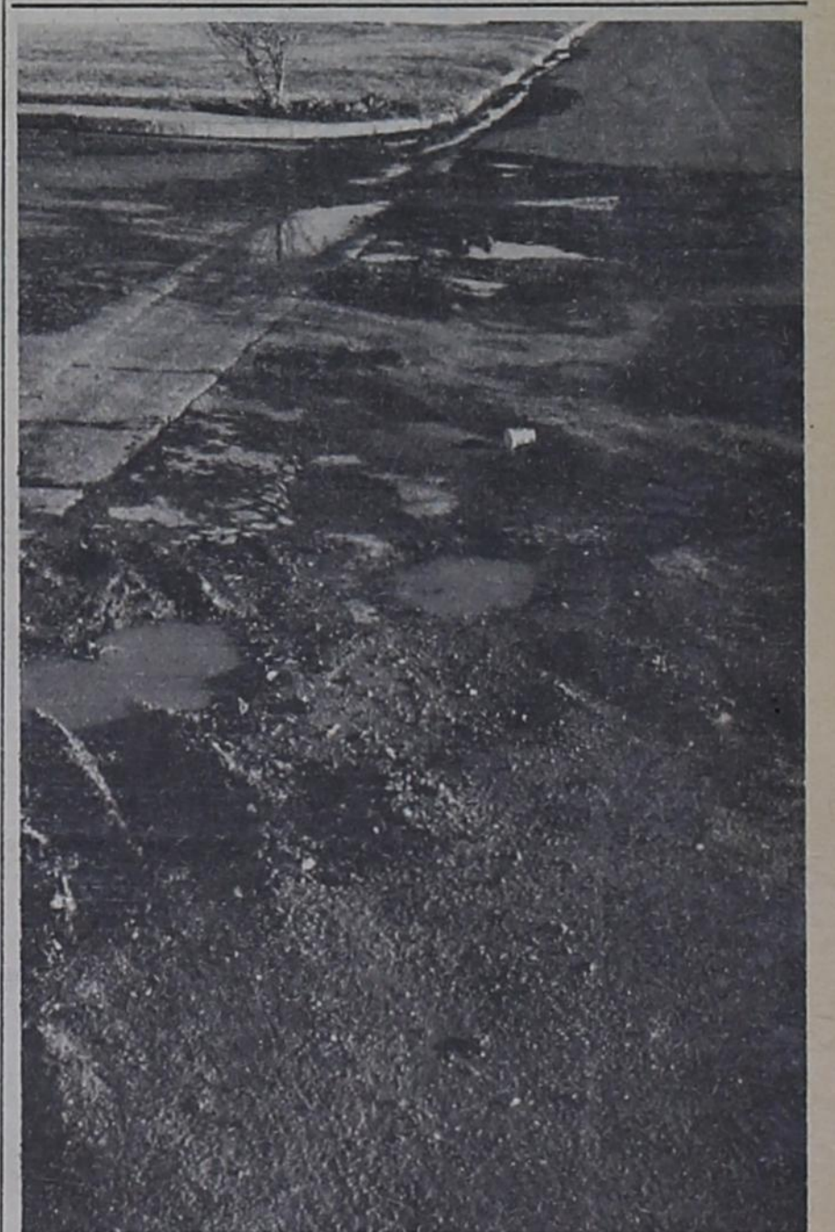
SNOW AFTERMATH --- The prolonged period of snow and ice on paved streets and highways had a tendency to cause holes to come in the pavement. An example is this intersection in Bovina's Ridgelea Addition. Members of Texas Highway Department have been busy the past few days repairing snow and ice-caused flaws on the highways in the county.
