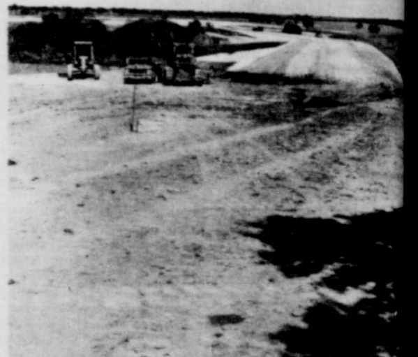
Construction of dam continues as dam height is increased.
