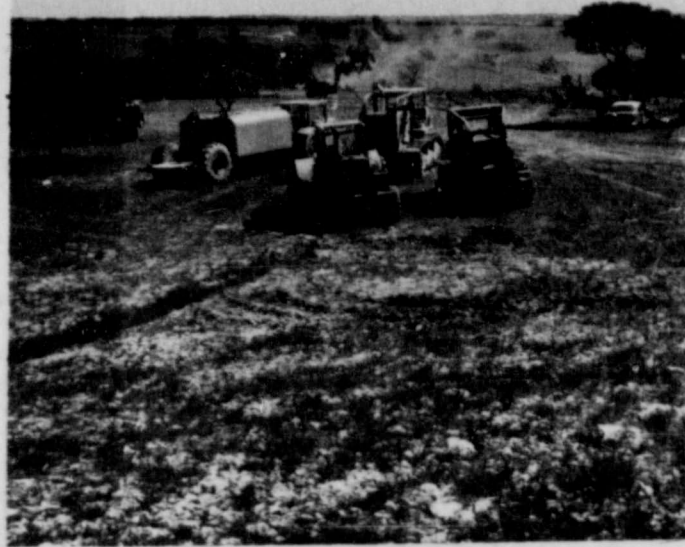
Contractor moved in and started clearing site last spring.
