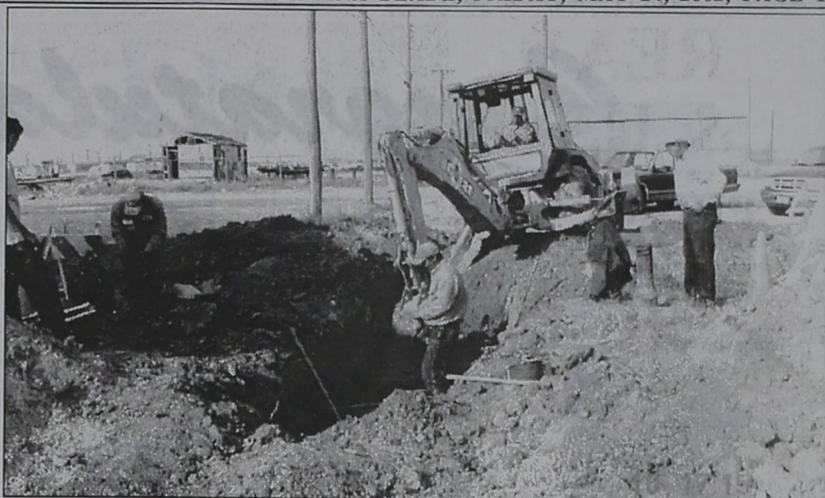
WORKERS TO REPLACE WATER LINE...Last Friday morning the water to the Gardner area was off until late Friday. Workers repaired and reconnected the break. The existing 2" line is scheduled to be replaced by a 6" line.
