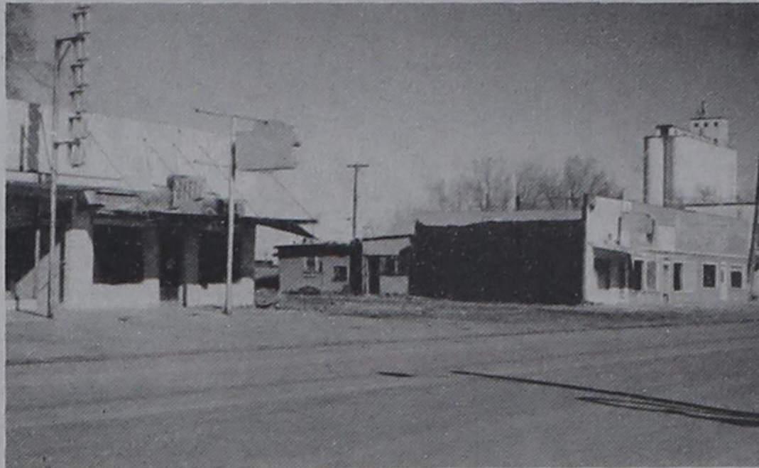
MORE BUILDINGS RAZED... A gap now marks a portion of Main Street in Bovina where a couple of old buildings were torn down this week. This is a part of the city's clean-up program.
