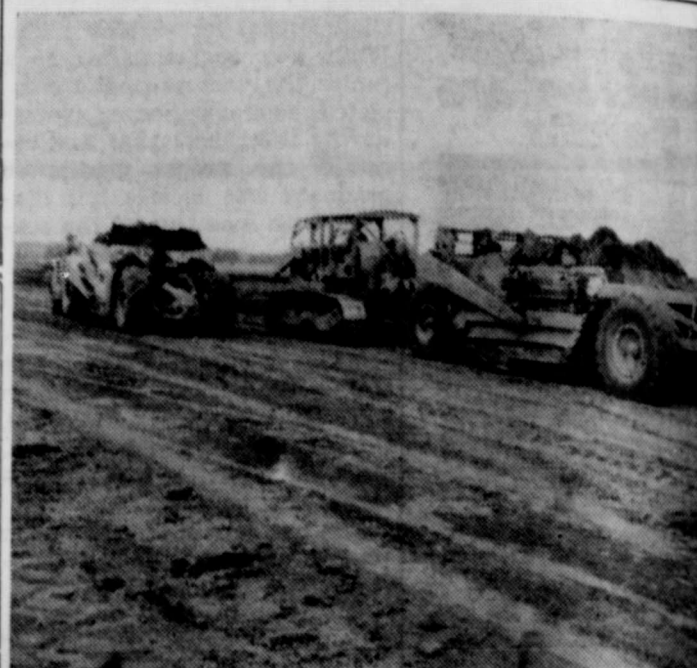
LAND LEVELING —Dirt moving equipment belonging to Brothers, Richland Springs, is shown here working on the Blackwell Ranch, Colorado River bottom land, at Regency and Carry-All are shown here moving dirt in a land leveling project.
