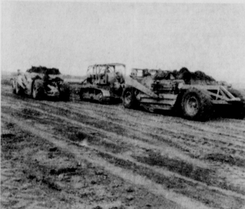
Here you can see our Cats and Carry-All equipment in operation moving dirt for Hollis Blackwell on Colorado River Bottom land at Regency. Step one in land leveling.
