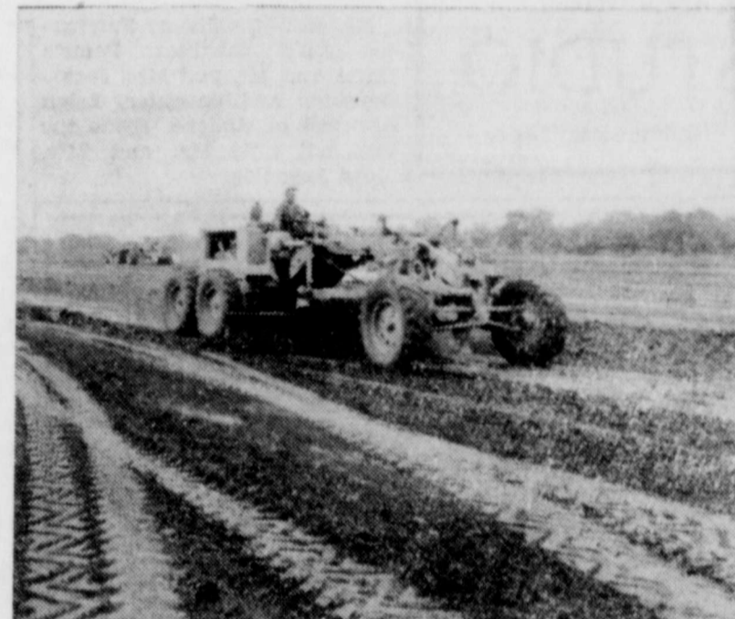
Step number two shows our grader-maintainer in operation on the land leveling project for Blackwell on the Regency project.
