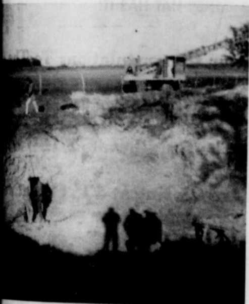
Excavating for Clear Well at Water Treatment Plant.
