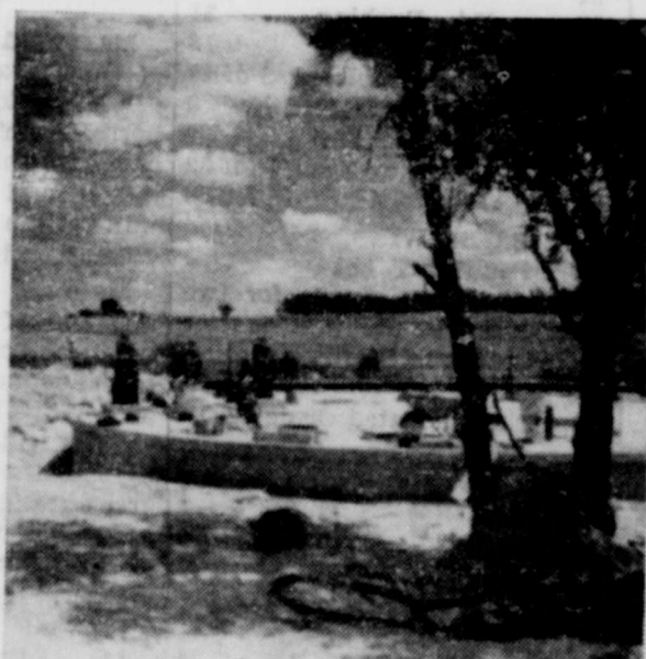
Clear Well with Top in place with construction moving ahead.
