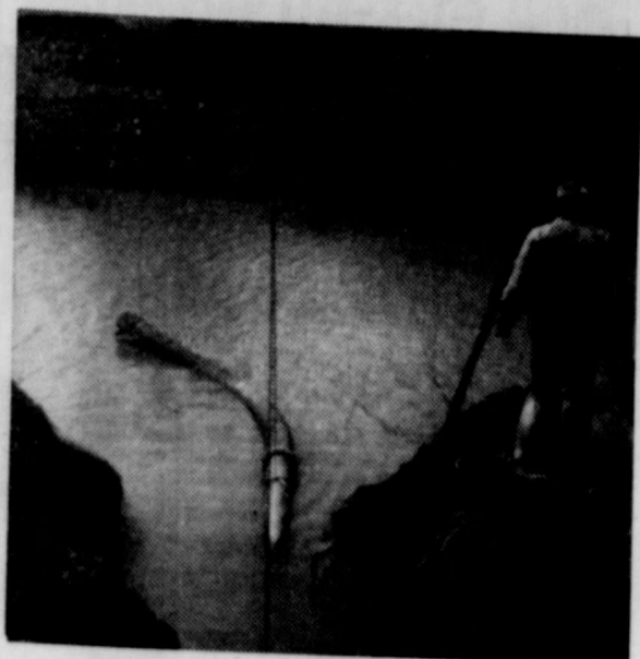
Installing Intake Line from Pump Station into the River.
