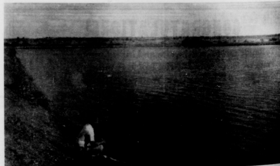
Another view of one Off-Channel Storage Reservoir showing the deep end in the background toward the right. The two Reservoirs have a capacity of approximately 120 acre feet; or 40 million gallons of water.
