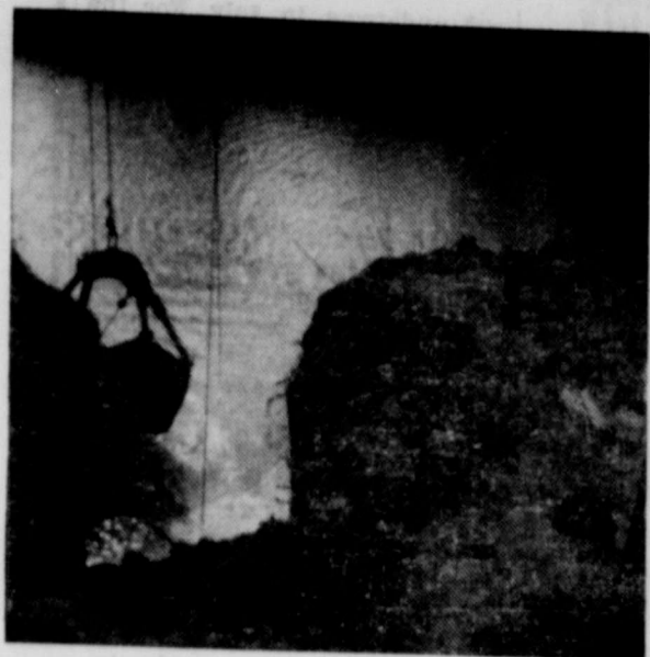
Cutting Channel from River to Pump Station Location.
