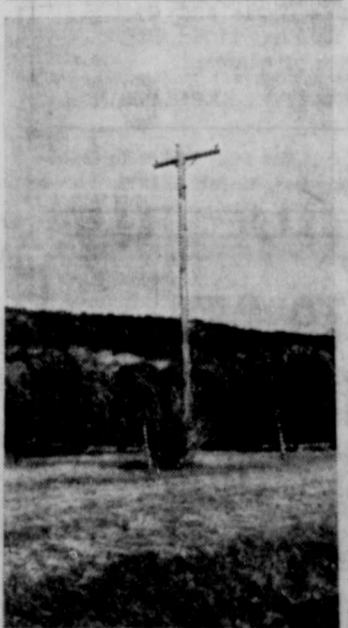
OLD STRUCTURE —This picture shows an average structure of the old power line from Lometa to Goldthwaite with a 12,000 volt capacity. This has been replaced with new power line from San Saba to Goldthwaite.
