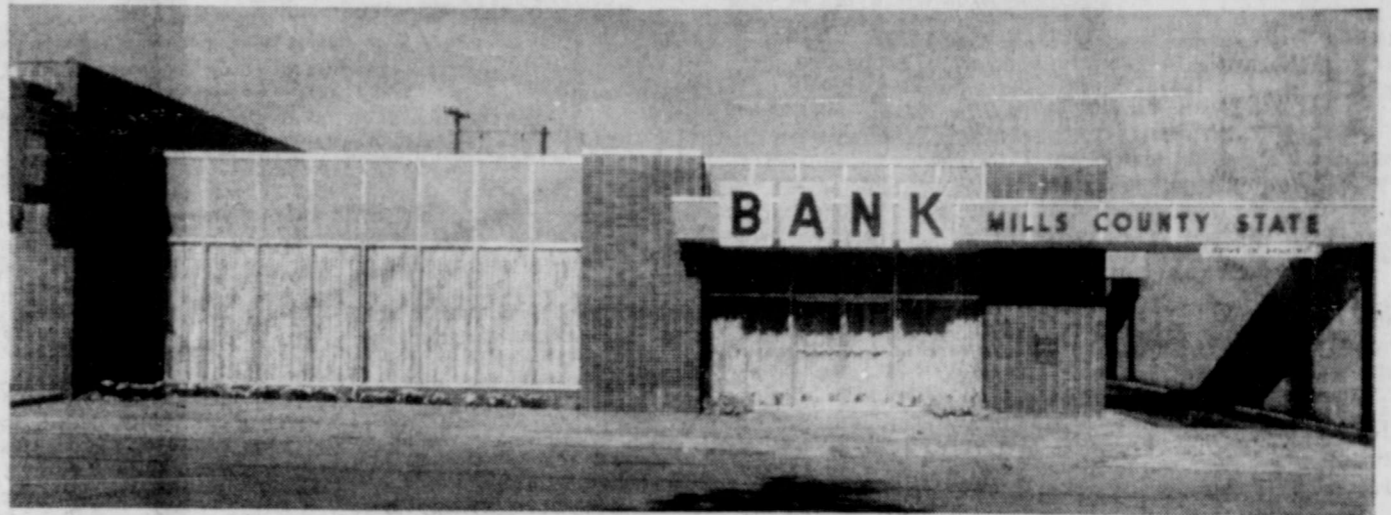
NEW BANK HOME IN QUIET OF MORNING —Here is the new home of Mills County State Bank, Goldthwaite, as it appears in the quiet hours of early morning before the bustling activities of the business day get underway. The new home was officially opened on Sunday, June 11, with a record open house attendance of 2,000 persons. —(Wicker Studio Photo)
