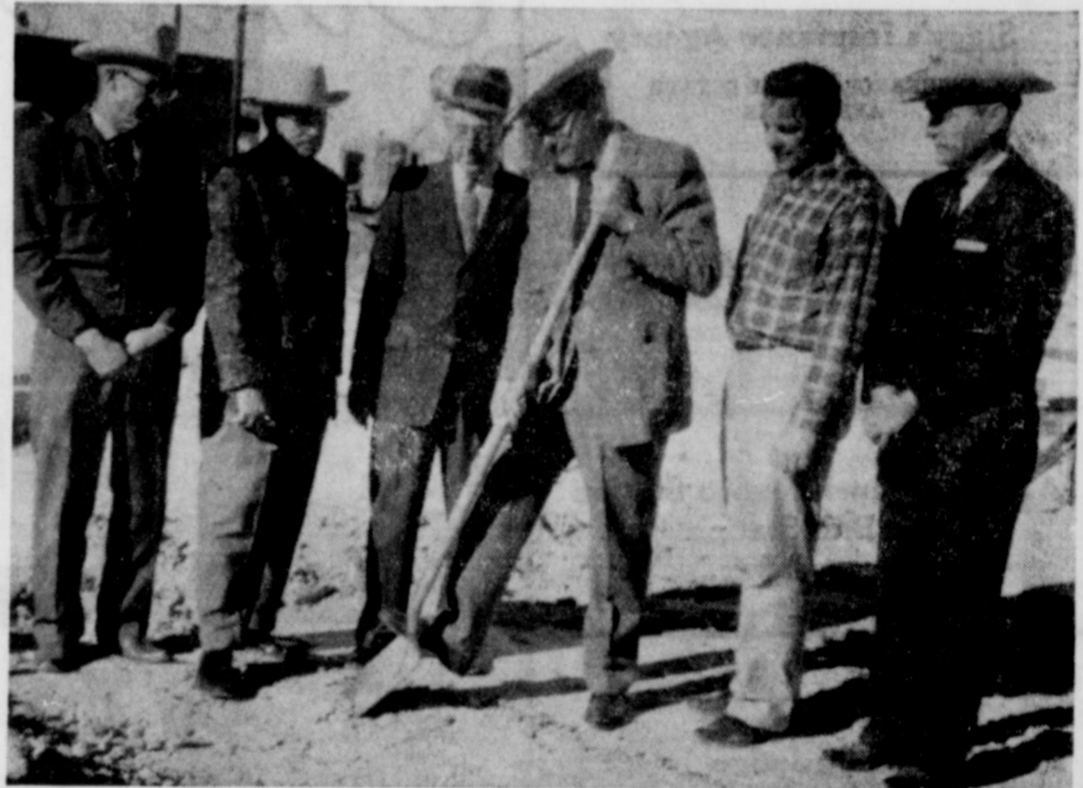
GROUND BREAKING FOR NEW BANK HOME—Warren P. Duren, president of Mills County State Bank, is shown here turning the first shovelful of earth last week Wednesday as actual construction on foundation for the new bank home got underway. Preliminary work of razing three old buildings which started ten days earlier had been completed. Looking on with Duren from left are: County Judge Cecil Egger; bank directors T. C. Graves and E. B. Gilliam, Jr.; general contractor W. H. Barsh and Mayor Y. B. Johnson, Jr. (Goldthwaite Eagle December 29, 1960.)
