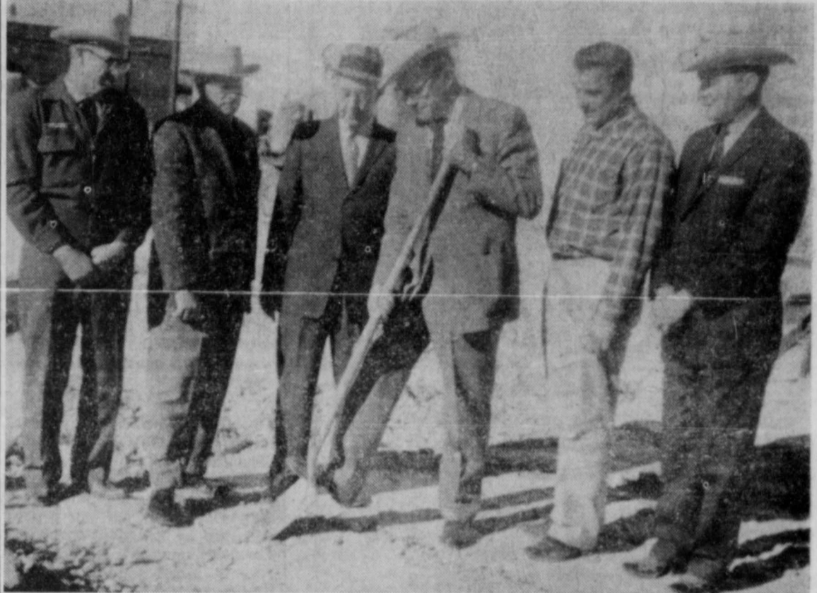
GROUND BREAKING FOR NEW BANK HOME —Warren P. Duren, president of Mills County State Bank, is shown here turning the first shovel of earth last week Wednesday as actual construction on foundation for the new bank home got underway. Preliminary work of razing three old buildings which started ten days earlier had been completed. Looking on with Duren from left are: County Judge Cecil Egger; bank directors T. C. Graves and E. B. Gilliam, Jr.; general contractor W. H. Barsh and Mayor Y. B. Johnson, Jr. Dr. J. C. Terrell, Stephenville, chairman of the board of Mills County State Bank, was unable to attend the groundbreaking. The new bank home will be located on the west side of the courthouse square, and represents an expenditure of approximately $110,000. New and modern in every detail it will offer drive-in bank service to customers and a community meeting room.
