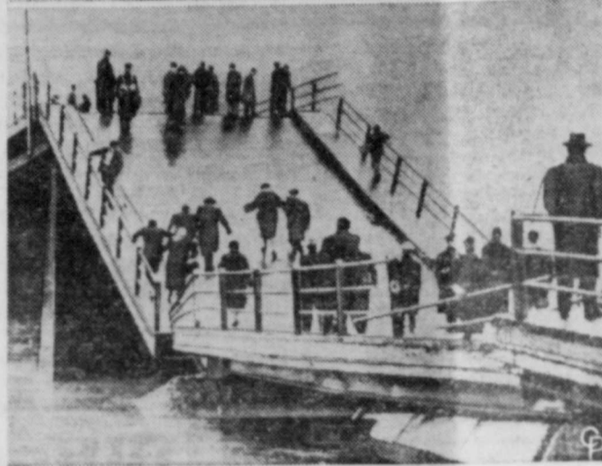
CHILE FACES MASSIVE EARTHQUAKE DAMAGE —Most of a building (top) is in the street in Concepcion, Chile, after a series of earthquakes left the city in ruins. More than 200 persons were dead and 100 missing in the devastated area, which stretched 500 miles south to Aneud. At bottom, residents of Concepcion cross a partly-collapsed bridge over the Bio Bio River. Torrential rains flooded stricken areas and new tremors were felt. Tidal waves from the earthquakes rolled across the Pacific to hit Hawaii and cities on the California coast.
