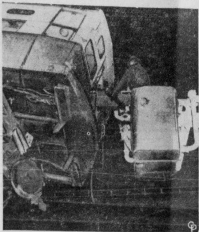
CHICAGO ELEVATED JUMPS THE TRACKS —A snorkel lift helps a fireman remove the injured from a teetering elevated train in Chicago. The engineer could offer no explanation for the sudden derailment as the train rounded a curve. Two of the 32 injured were in critical condition but passengers could be thankful that the two-car train had not plunged to the street.
