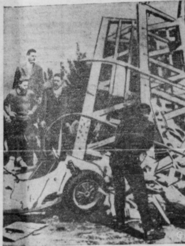
SEVEN DIE AS BRIDGE FALLS ON RACING CAR —The remains of British driver Chris Threlfall's racing car lies amid the wreckage of an overpass which collapsed on top of it in Aix-les-Bains, France. Threlfall, 30, was killed instantly and six persons standing on the span also died. At least 50 persons were injured as the spectator-jammed overpass fell. Four drivers behind Threlfall were able to brake to a halt before they hit.
