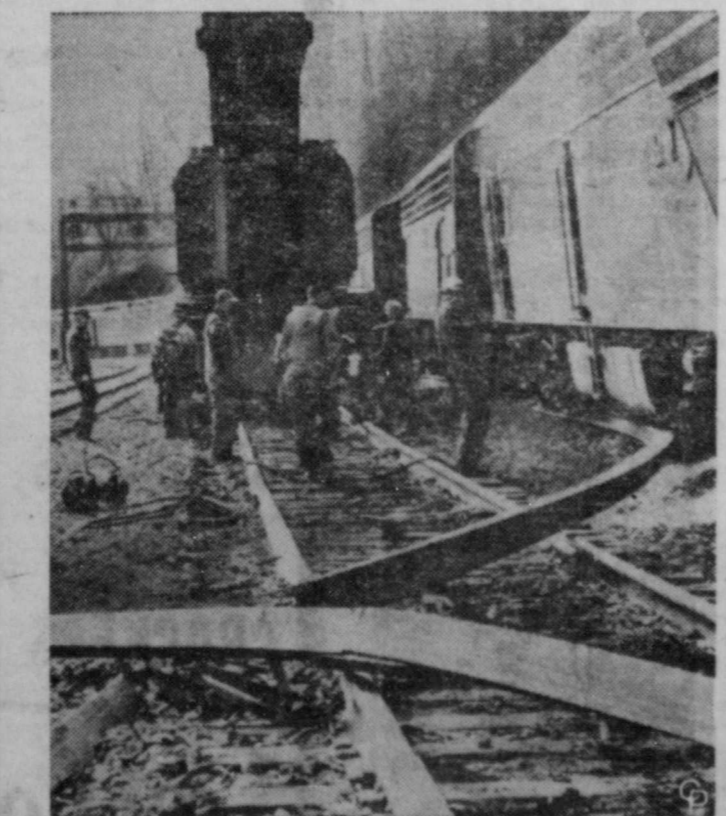
EIGHT HURT IN DERAILMENT —Salvage crews of the Baltimore and Ohio Railroad work amid twisted rails and damaged coaches in an effort to put back on its tracks the crack National Limited after it was derailed near Newburg, W. Va. Eight persons were hospitalized and many others shaken up.
