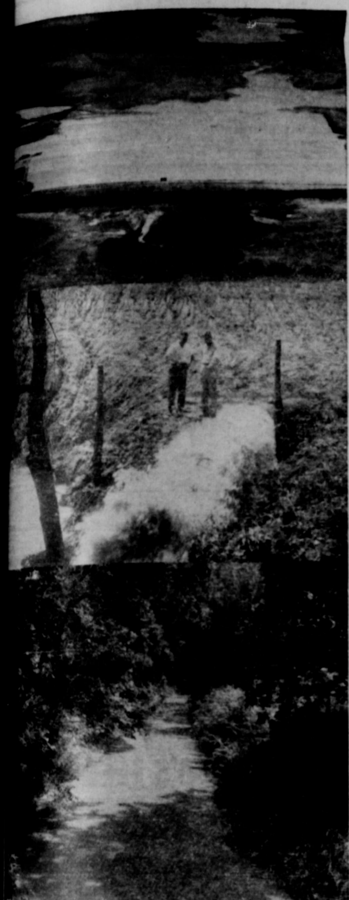
TOP—Flood water held behind retarding structure. CENTER—Discharge from drawdown tube. BOTTOM—Stream is about one-third full but is not overflowing.
