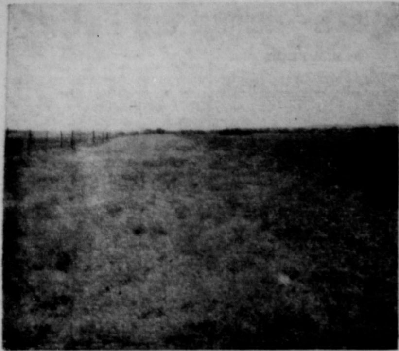
WATERWAY DEVELOPMENT —Here is an ideal picture of a grassed waterway used for terrace outlet on the Elzie Ault farm 15 miles southeast of Goldthwaite. Waterway is sodded to Bermuda grass.—(SCS Photo)
