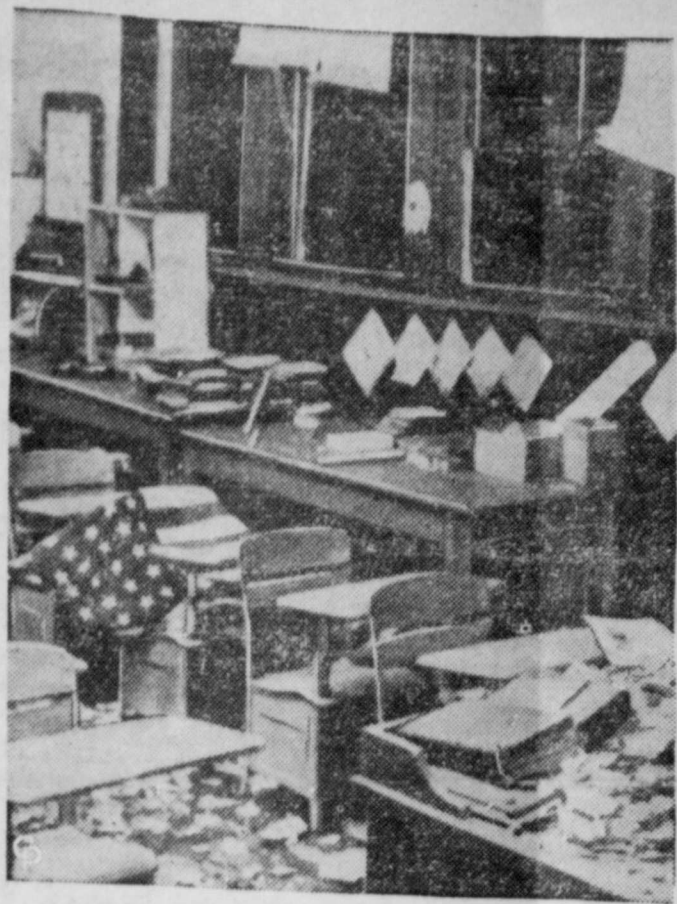
DYNAMITED SCHOOL ROOM —An American flag is draped over a chair in one of the less damaged rooms of the Osage Junior High School at Morgantown, W. Va., after the building was ripped by two dynamite explosions. The school has been considered a model in the peaceful integration of students.
