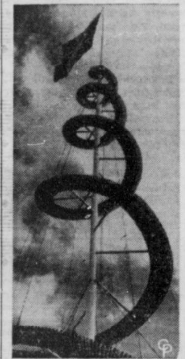
PIPING UP —Stretching 165 feet into the air is this spiral tower in the Belgian section of the Brussels World Fair. The tower was built of 1,270 pipes, which grow shorter in length as they reach up to the top.
