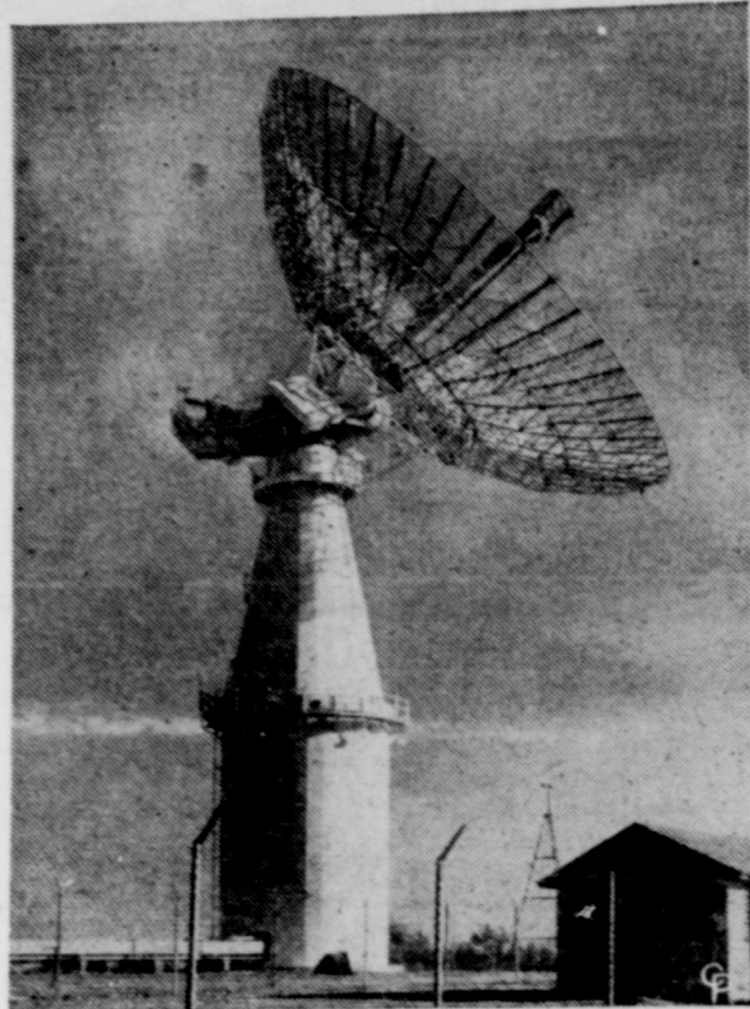
NEW RADAR RESEARCH TOWER —This radar "Sherlock," which has already tracked Sputniks No. 1 and 2, will be used to check future Red earth satellites. The tower rises 90 feet above Westford, Mass. It will be used by the U. S. Air Force, the Naval Research Laboratory and the Defense Research Board of Canada in their Project Vanguard program for International Geophysical Year.
