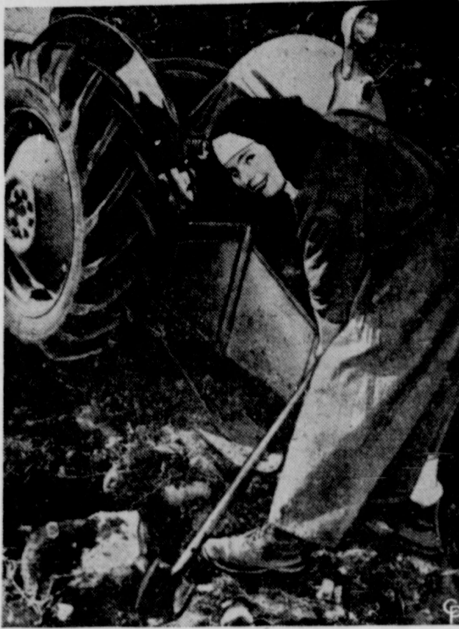
SISTER INGRID, Sweden's first native Dominican nun, is shown at work helping clear the land where the first monastery is that country since the 16th Century is under construction at Sodra Sandy. Her task is to clear ten acres of farm land. (International)
