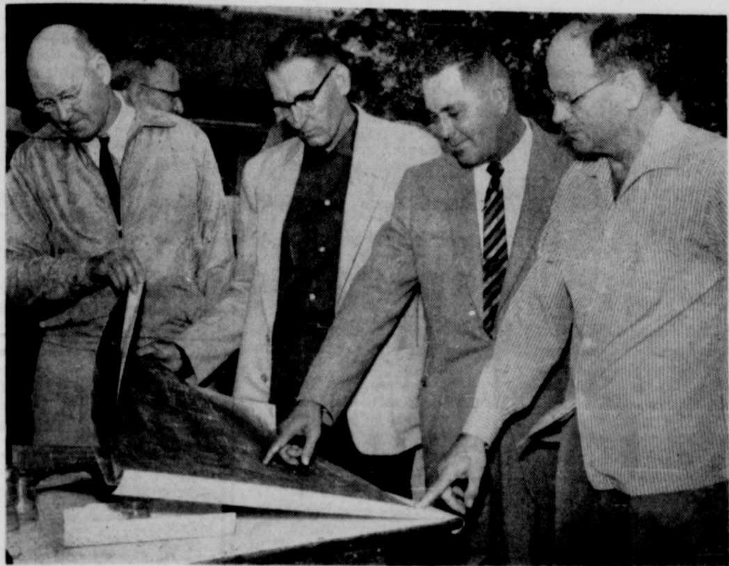
GROUND BREAKING—Shown in this picture are Rev. M. O. Childress; Loy Long, former mayor of the City of Goldth-
