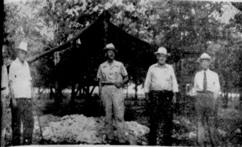
SHAFT—This newly opened shaft with windlass and tarpaulin shed has been dug to depth which runs 20 feet below surface. Left to right, George Ellis, Mullin mail carrier; W. H. Hester, owner of Dry Pond; J. A. Hester, Goldthwaite wool and mohair dealer; Charles T. Goldthwaite Eagle editor, and Ernest Jones, Bulletin editor.
