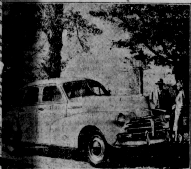
Over-all simplicity and massiveness of the new, 1948 Chevrolet is well shown in this three-quarter view of the Fleetmaster Sport Sedan. Fenders, body and door panels all blend; and the crease moulding, below the new, wider than that used in previous models. Note the new T-shaped center bar on the radiator grille.
