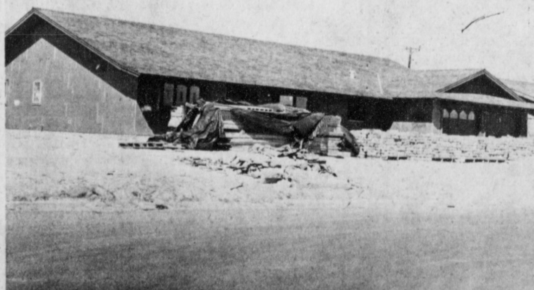
NEW CONSTRUCTION . . . . . This is only one of several new homes that are being constructed in Muleshoe at the present time. Excellent winter weather has permitted the work to go at a rapid pace this year. This new home is located on 20th Street in Richland Hills.
