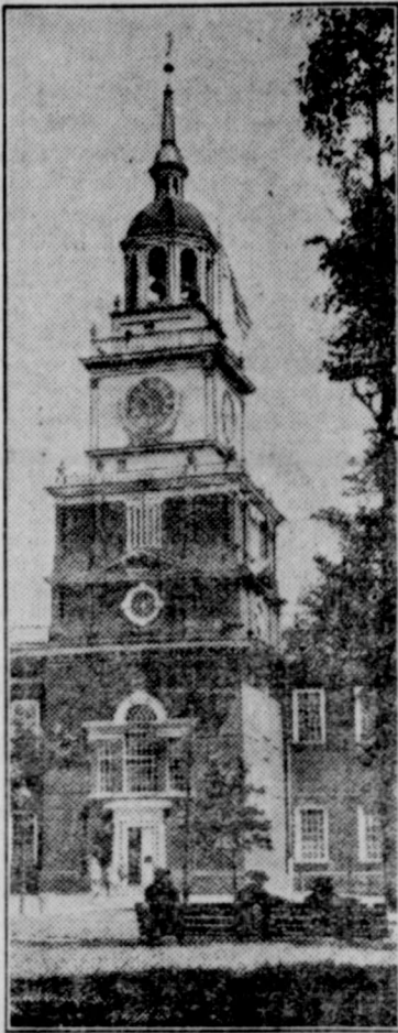
Picture taking is more fun when you choose a specialty and master it. Architectural pictures—such as this shot of Independence Hall, model for many a county court-house—make up one of many fascinating fields
