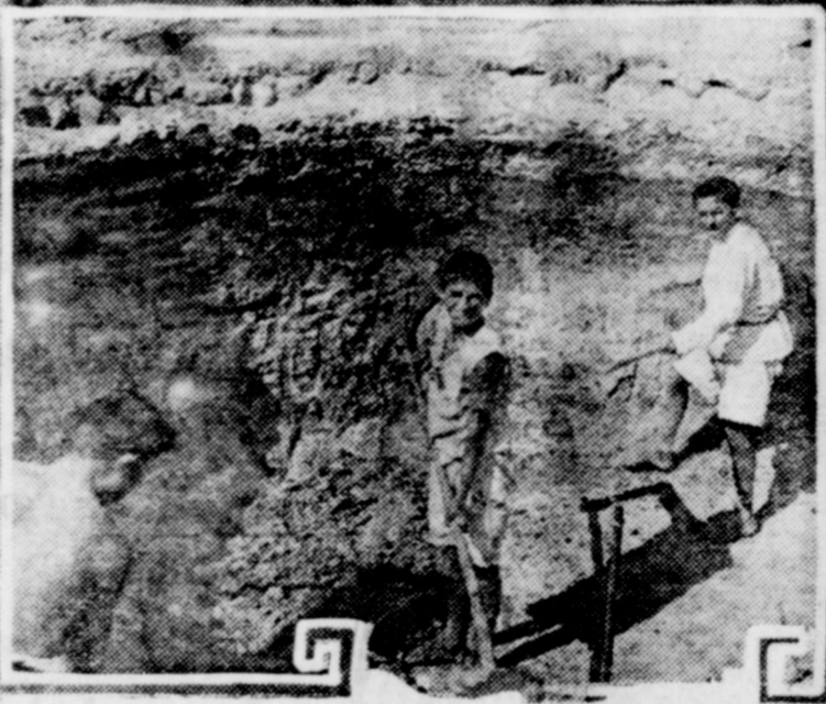
The first silos in the Russian Caucasus have been built by Near East Relief at its Agricultural Training School in Leninakan. In order to save time and money they were placed below ground. The work was done by orphan students of the school.
