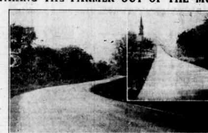
the asphaltic or bituminous mat in their gigantic task of taking the American Farmer out of the mud. Smooth and durable, bituminous mats like those illustrated, are proving far more economical than gravel when investment and maintenance are considered. Their cost ranges from \$1,000 to \$5,000 a mile. The high type asphaltic surfaces are used extensively on the main arterial highways and city
