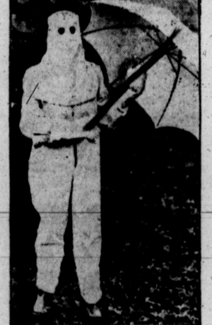
London's firemen are now outfitted with asbestos umbrellas as well as with the regulation asbestos suits. Thus they are protected from falling embers and are able to approach more closely to a burning structure.
